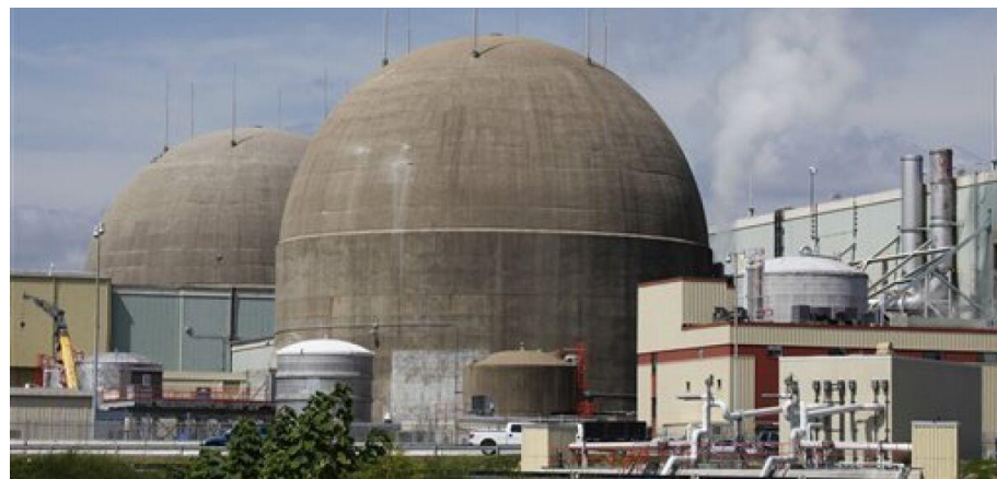
Automatic Protective Relay: 110823, Mineral VA
