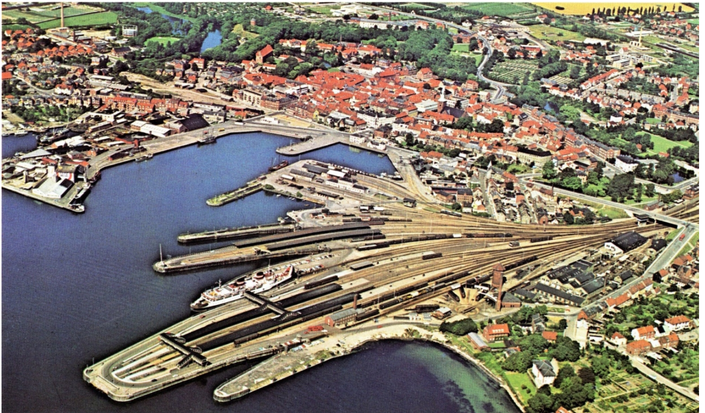
An old postcard of the ferry port dominated by railway tracks. The DSB roundhouse
