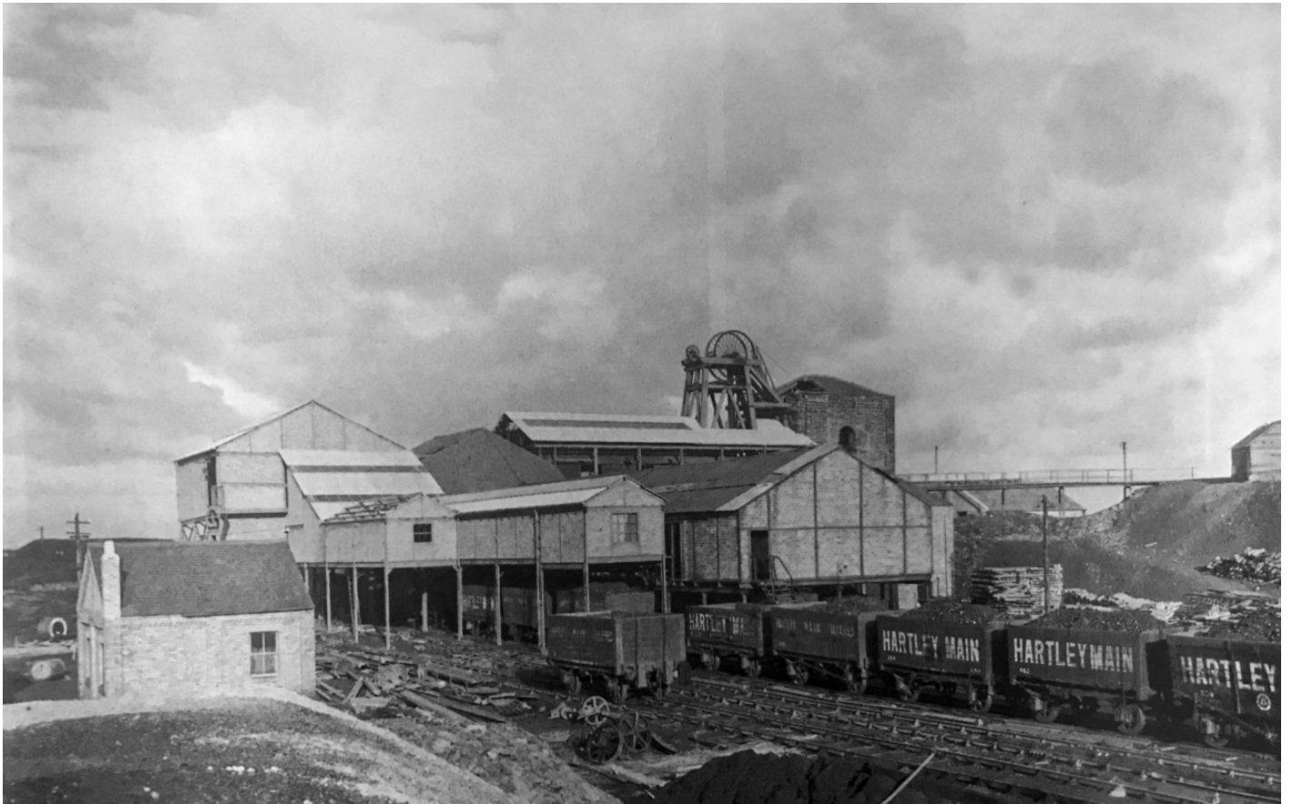
Amelia Pit Shankhouse Northumberland c 1938. Hartley Main was the company that operated many of the collieries on the Delaval land and beyond.
