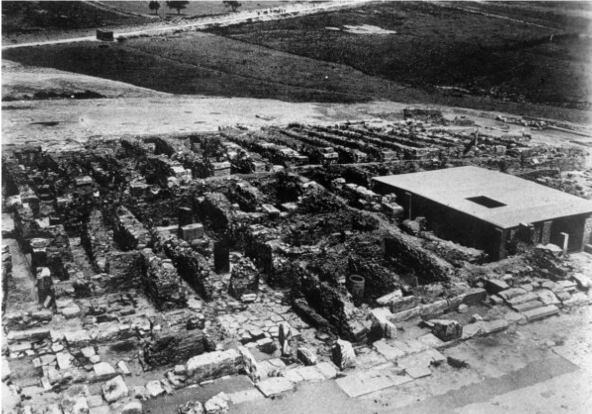
Before – a roof arresting the decay.
