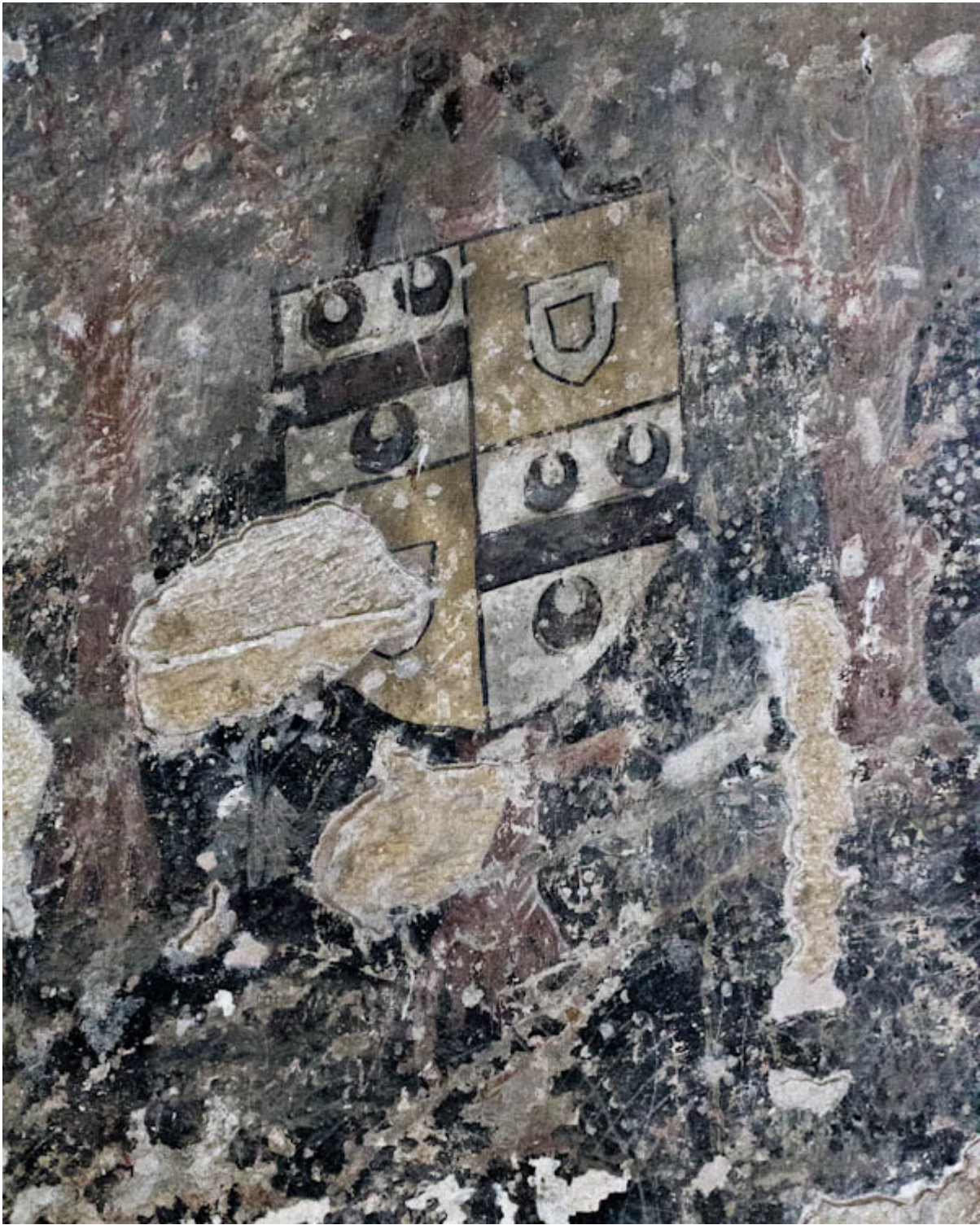
Original painted plaster in the great hall of the medieval tower
