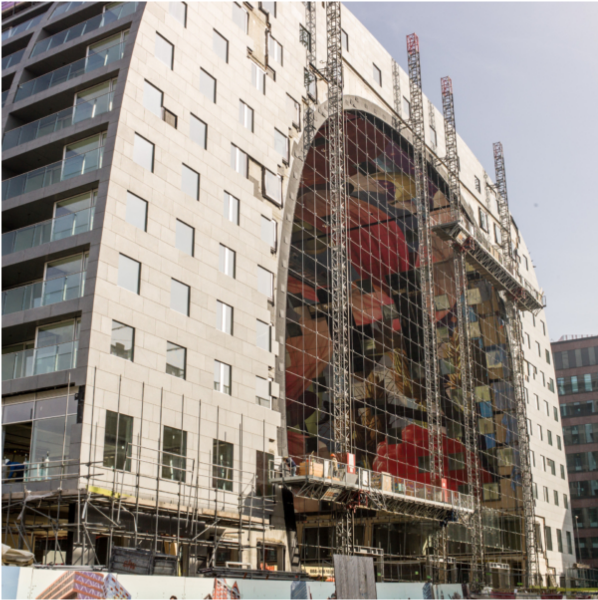
Building the new Market Hall
